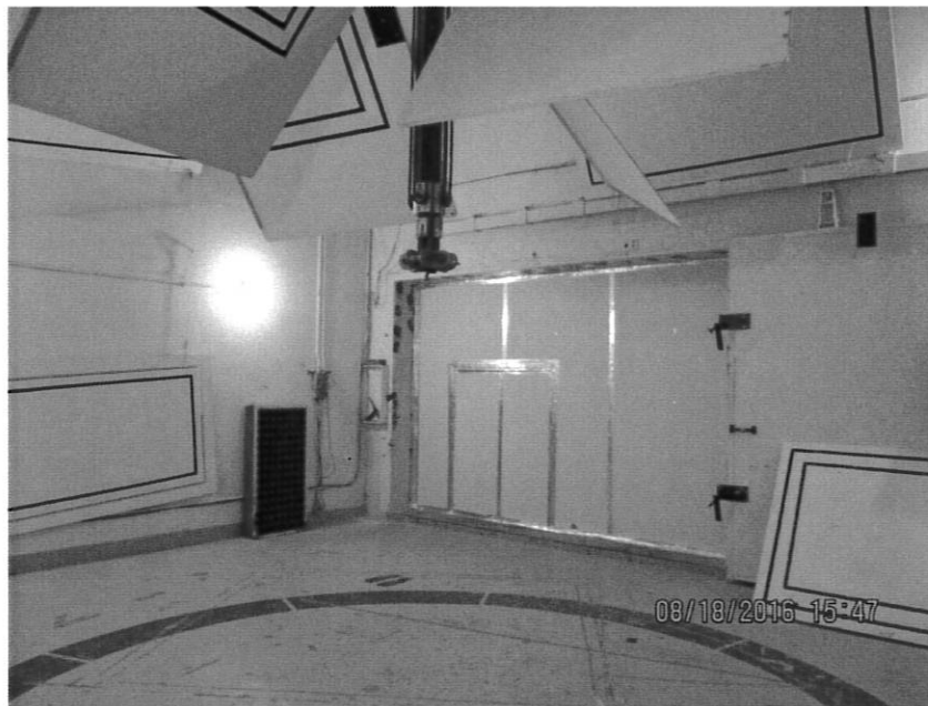
Figure 1. Filler wall with support structure built to accommodate 1418 mm x 1138 mm single pane wood window with the opening closed and finished with glass fiber and 2 layers of gypsum board on each side.
