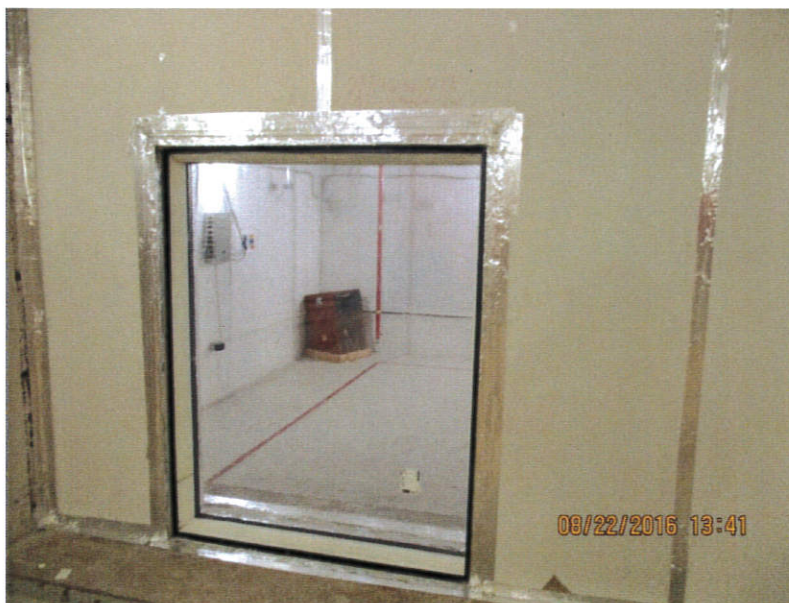
Figure 5. 1496 mm high x 1196 mm wide Magnetite Framing System was installed 100 mm away from the 1457 mm high x 1178 mm wide double pane aluminum window.
